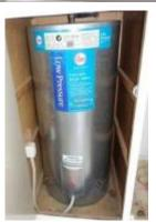
• There is no over-flow tray or over-flow does not flow to an exterior drain.
