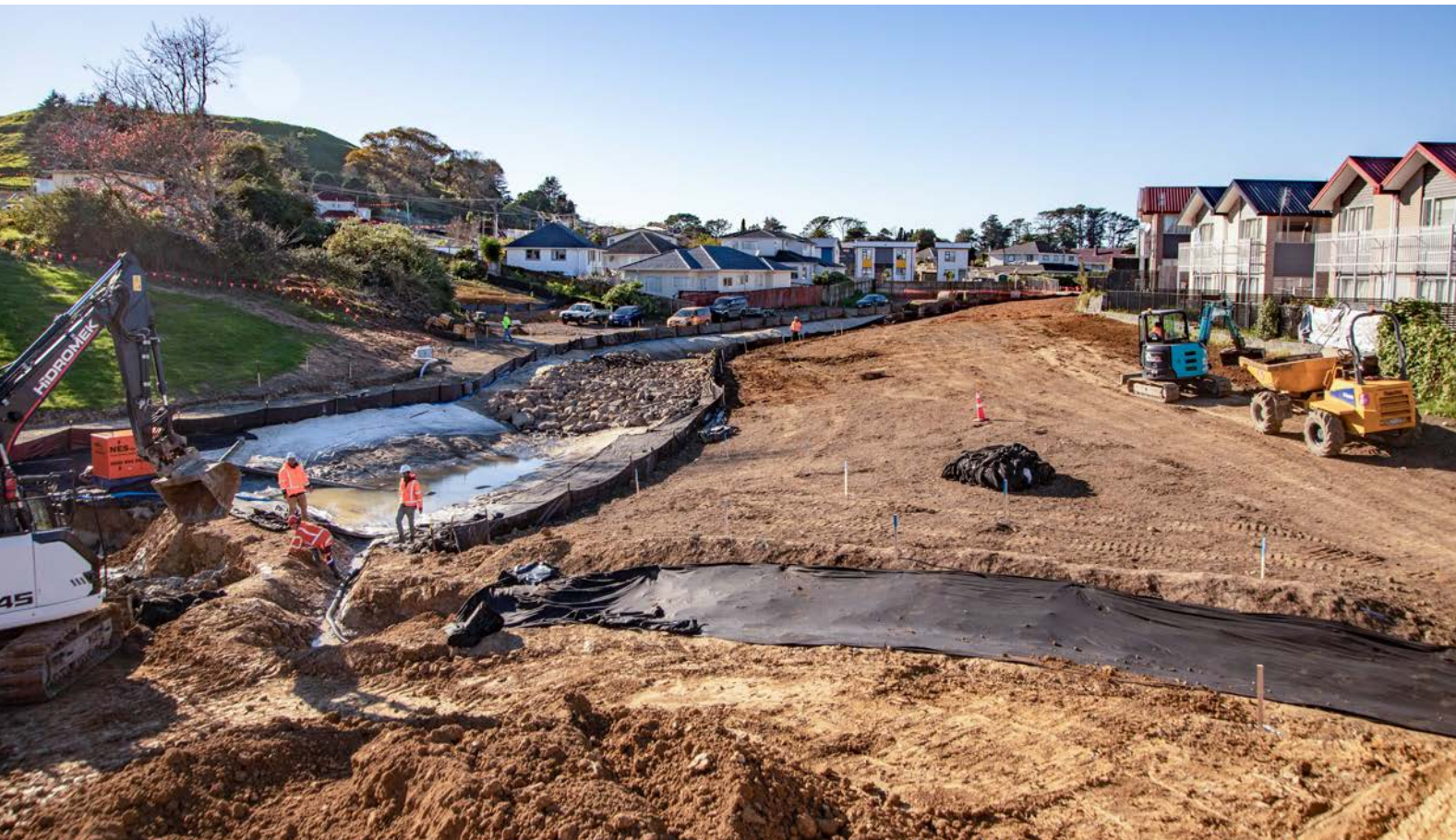
Location: Freeland Reserve earthworks, Mt Roskill, Auckland
