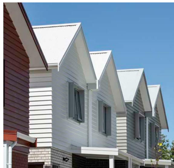
Location: Waterbank Crescent, Waterview, Auckland
